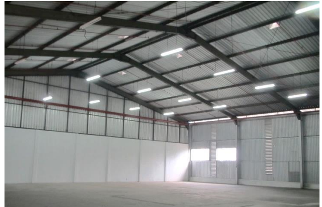
Warehouse internal view
