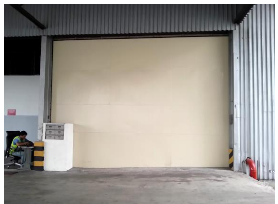
Warehouse entrance 2 external view
