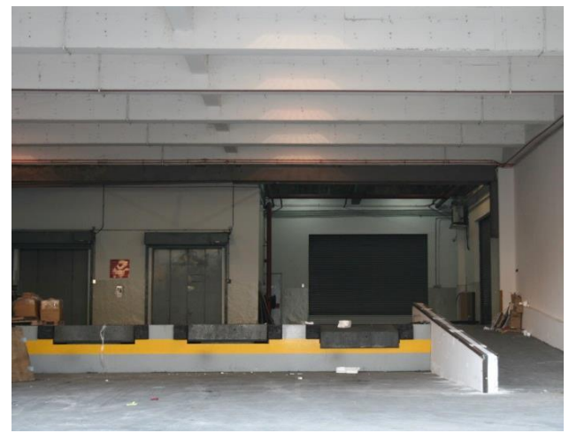
Loading area with 4 loading bays
