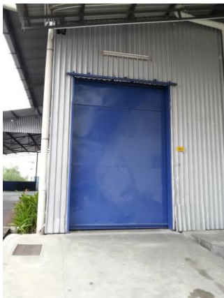
Warehouse entrance 1 external view
