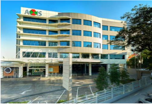
Axis Business Park (Block C)
