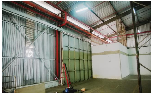
Warehouse entrance 2 internal view
