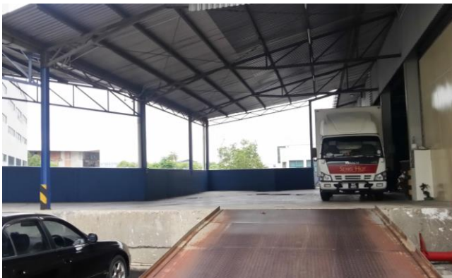
Loading ramp to warehouse entrance 2
